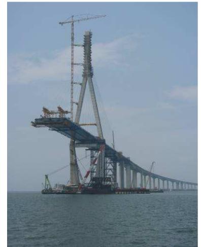
Incheon Cable-Stayed Bridge under construction in South Korea.
