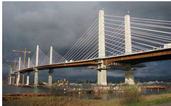
The Golden Ears Bridge over the Fraser River near Langley, BC nearing completion in November 2008.
